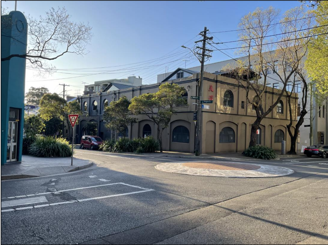
Figure 2: Site viewed from intersection of Meagher St and Balfour St
