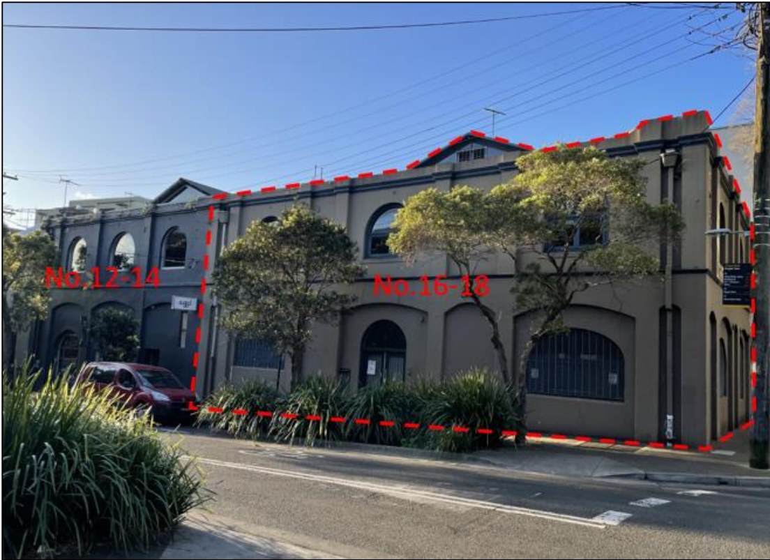
Figure 4: Site viewed from Meagher St
